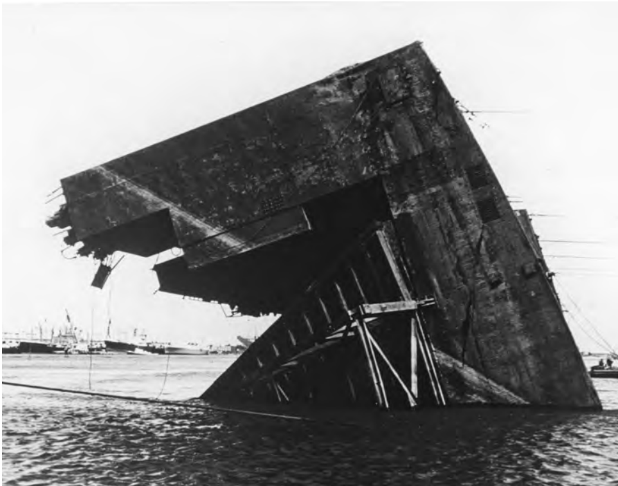
The floating drydock AFDM-2 set off a complex salvage job when it capsized and sank in the Mississippi at New Orleans. Here it is partially righted after 4,000 tons of mud had been removed.
