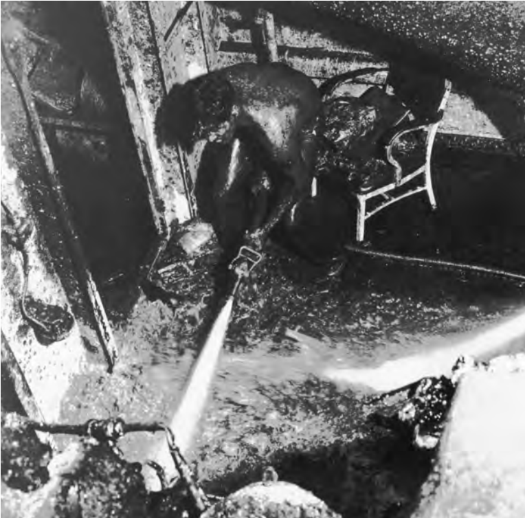
It's a dirty job! A salvor with a fire hose washes mud out of the Rajah Soliman to lighten the ship.
