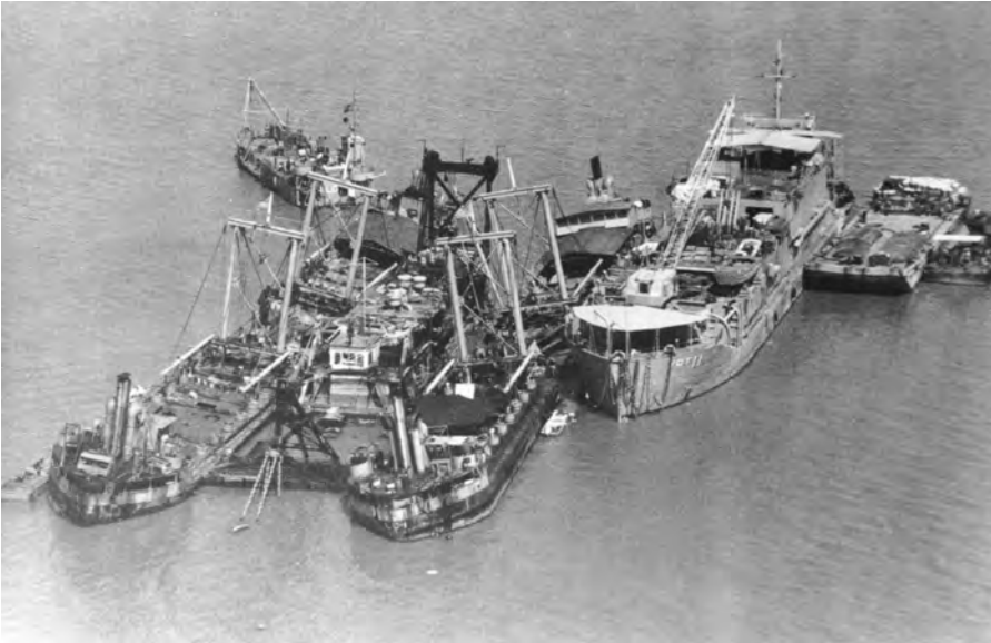
Four lift craft, assisted by YDT-11 , YLLC-2 , and various other craft, raise the dredge Jamaica Bay near the Ninth Infantry Division base at Dong Tam, Vietnam.
