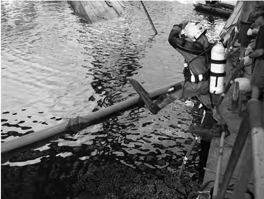
A Navy diver in a contaminated-water suit enters the Industrial Seaway in Gulfport, Mississippi, for clearance operations.
