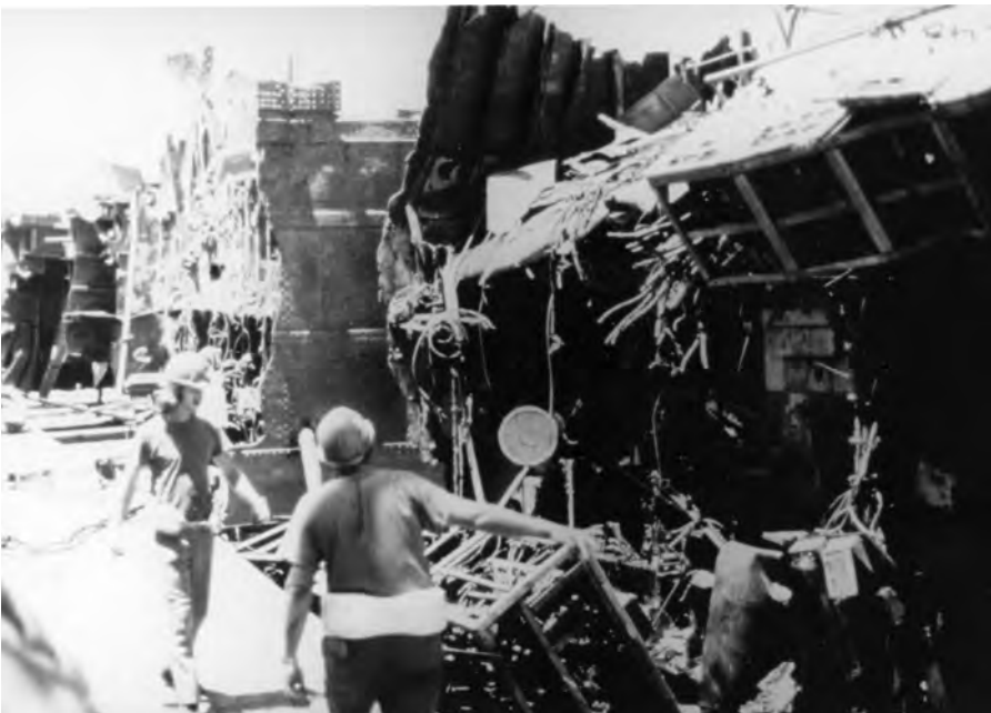
Sections of Mackenzie are lined up on a barge after having been lifted out. All of the cutting was performed by divers working underwater in near zero visibility.
