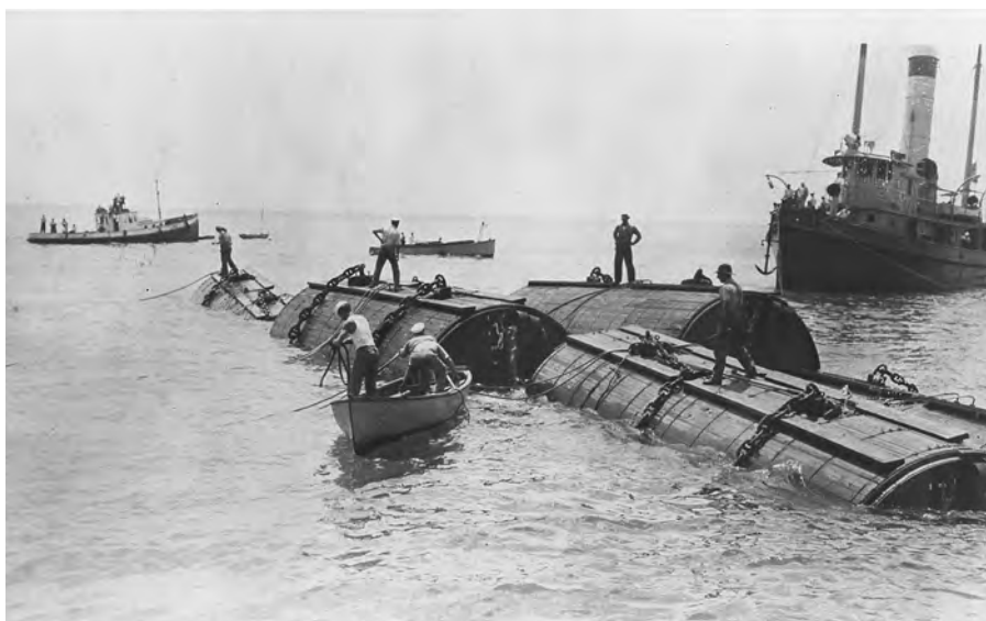
The final lift of the submarine F-4 was made using these submarine salvage pontoons designed by Naval Constructor Julius A. Furer.
