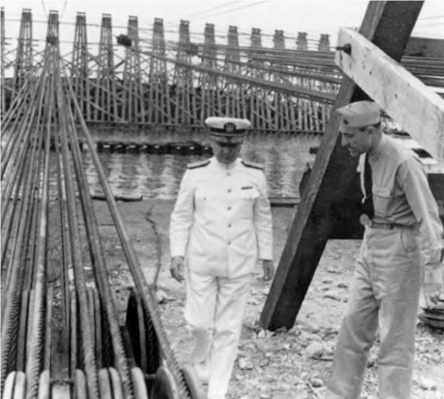
Rear Admiral Furlong (left) and Captain Francis H. Whittaker inspect the purchases used to haul Oklahoma upright.
