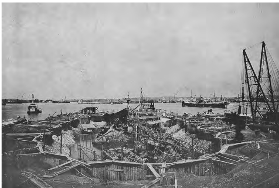
Earth-filled cofferdams 54 feet in diameter provide access to the wreck of the battleship Maine on the bottom of Havana harbor.
