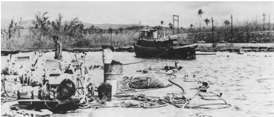
Salvors working in Guam after Typhoon Pamela undertake a variety of tasks. Top: Pumping out a sunken torpedo retriever. Center: Using a fire hose to wash away the bottom from under a stranded barge. Bottom: Rigging beach gear to refloat a grounded tug.
