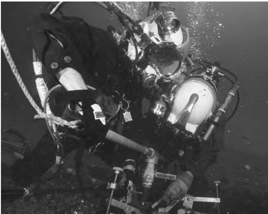
Navy divers hot tapping Mississinewa's tanks.
